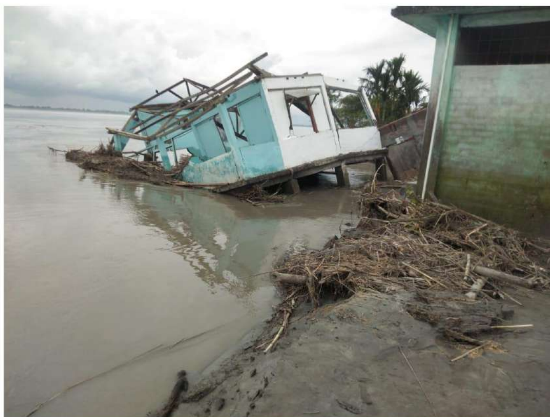
Picture-1: A broken house at the bank of river Lohit
